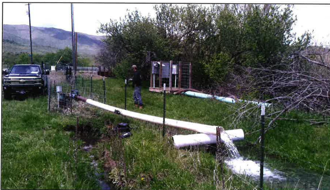
Figure 2: Well being pumped with flowmeter mounted on 6-inch PVC pipe about 12 feet downstream of the well head. PVC pipe was temporary for the flow measurement.
