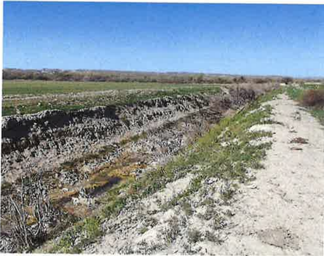
"South drain" looking east
