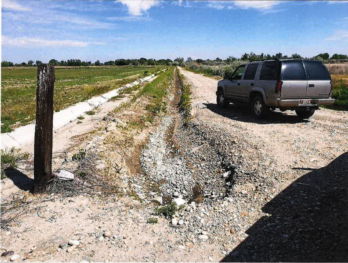
Dirt ditch that takes water to the back section of the property on the east side.
