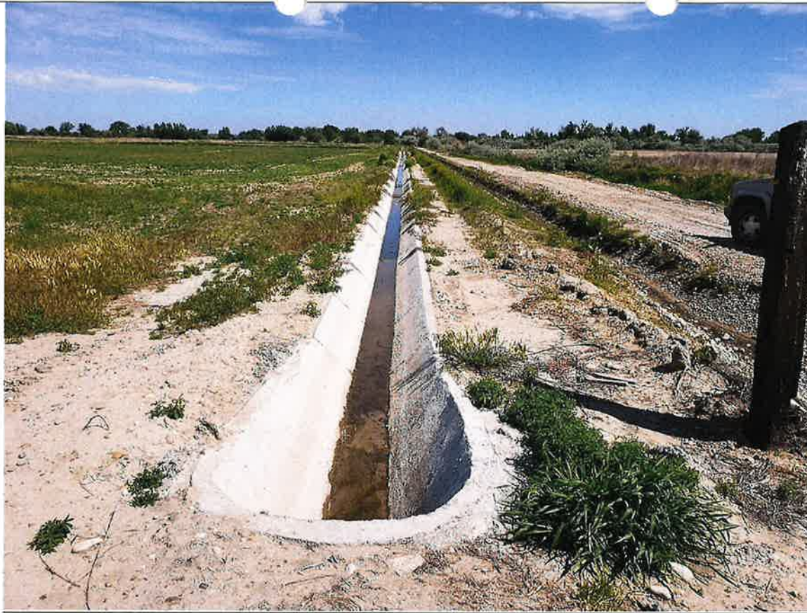
Concrete ditch that takes water along the roads and back into the Boise River at the north section of the property.
