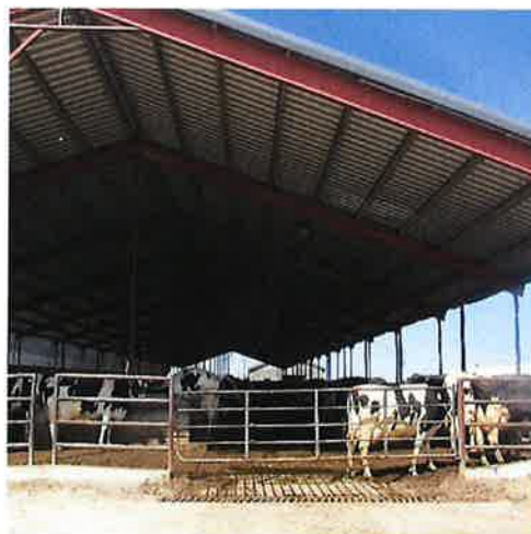
Barn near dairy #1
