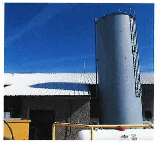
20,000 gallon storage tank at dairy #1
