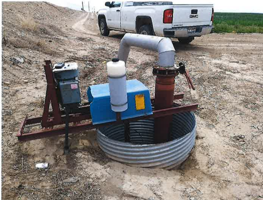
Figure 1 The POD is a Parma pump driven by a 10 hp Marathon Motor. Pump rpm is 868. Lift to first open discharge is approximately 40 ft.
