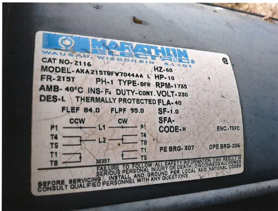
Figure 2 The specs for the electric motor. Motor speed is 1735 rpm w/ a 6" pulley. The motor pulley drives the 12" pump pulley using a serpentine belt. Pump rpm is half that of the motor.
