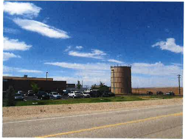
North side of facility and water tank
