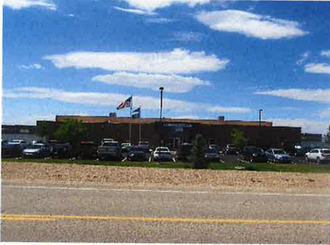
Overall view from the front of the facility
