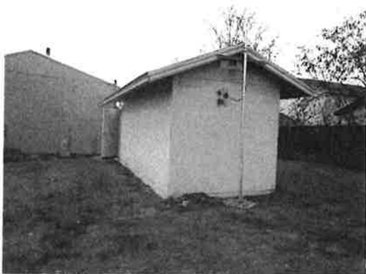
Elk well house (fenced well lot)
