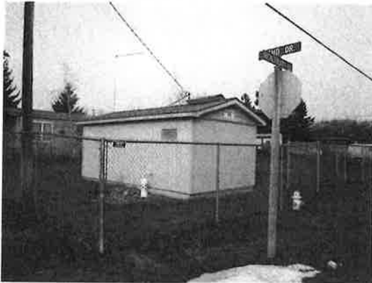
Huckleberry pump house
