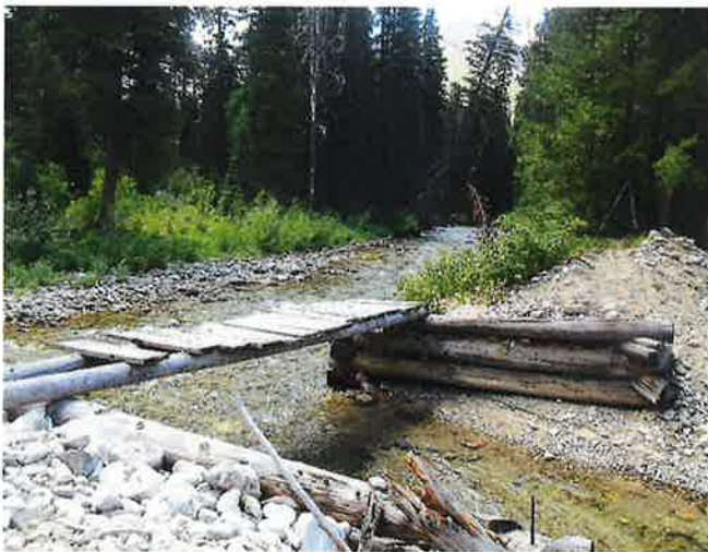
Main channel of Loon Creek (left), diversion to reservoir (right)
