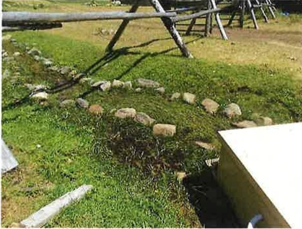
Channel downstream of turbines
