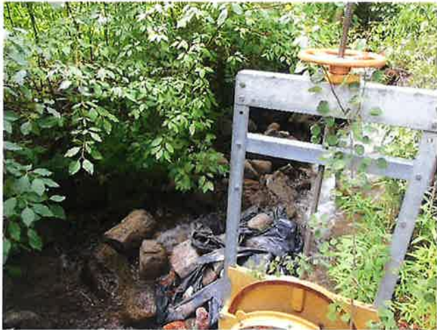
Headgate and point of diversion from Deer Creek
