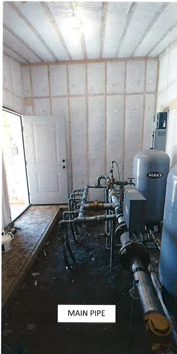
WATER SYSTEM PRESSURE TANKS
