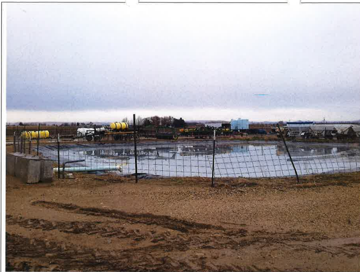
Fire Protection Storage Pond. Pond capacity is 1.4 AF with calculated evap of 0.6 AF.
