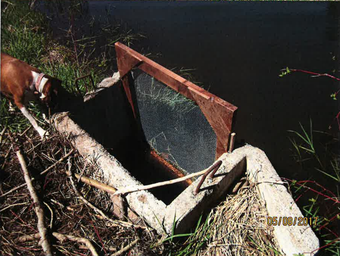
Point where water is diverted to the ponds. A screen is in place to control fish from going into the pond and debris.
