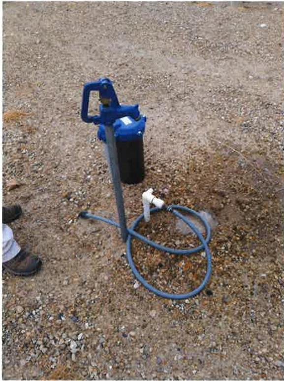
Figure 1 The well w/ hydrant. The hand line used to water the 1-acre field was run from the hydrant.
