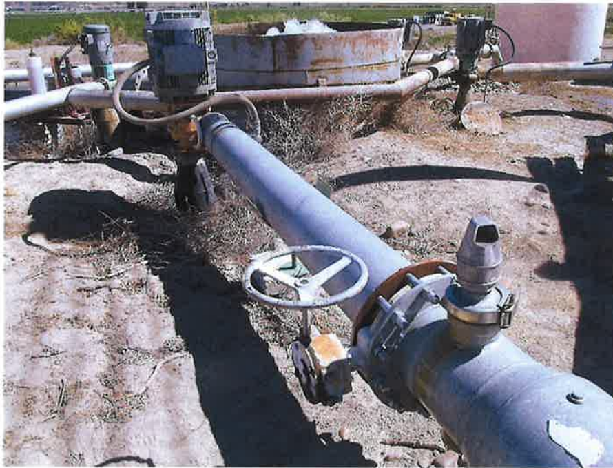
Photo 1: Diversion from Shoofly Creek
