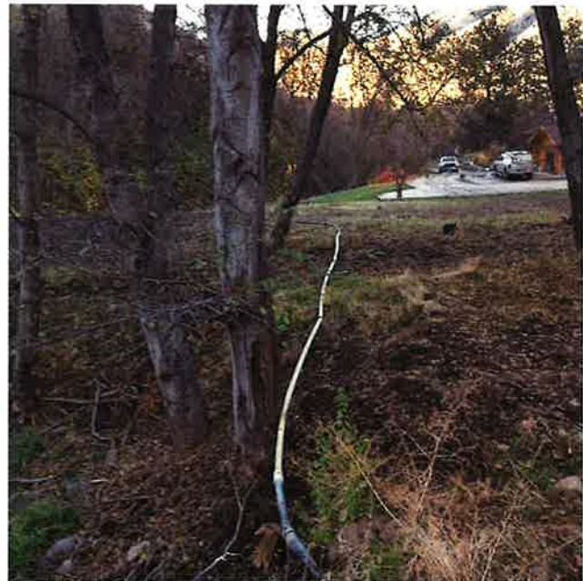
Spring 4 water line to portion of Irrigation Place of Use & pond. Pond to Right of vehicles.
