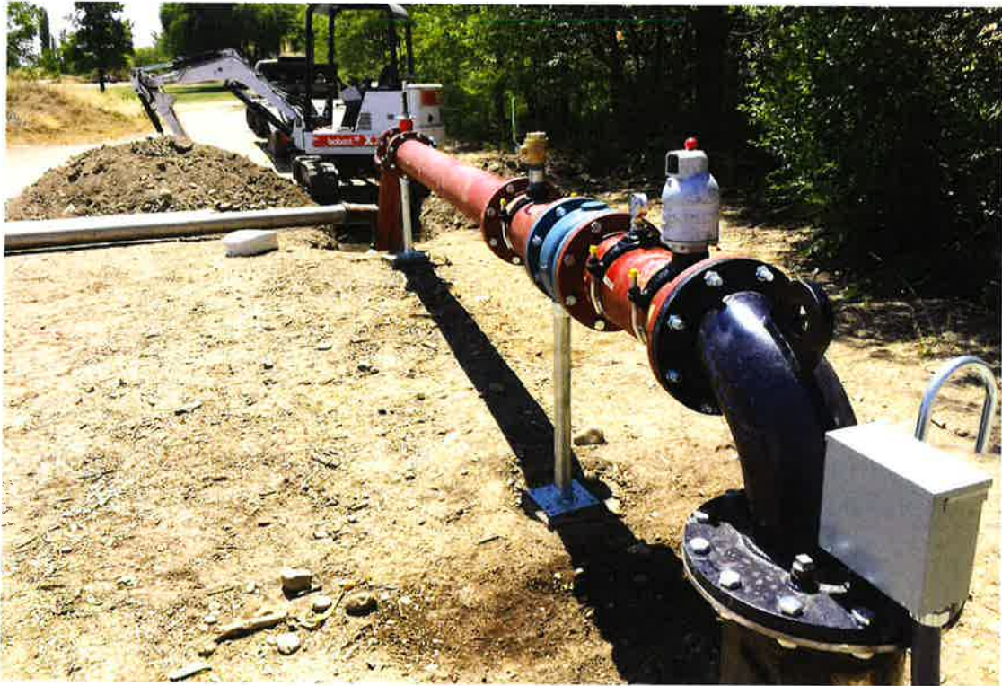
Well 2 and discharge piping. Mechanical piping appurtenances (from right to left) include discharge elbow, air/vacuum valve, pressure gage, check valve, 2-inch ball valve for winterization, straight spool for future flow meter, pressure relief valve, and butterfly valve (not visible, but located immediately past pressure relief valve).
