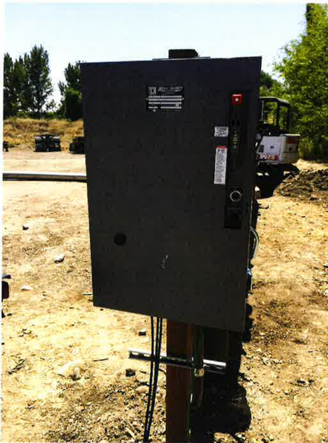
Well 2 Pump Panel. Pump is constant speed.
