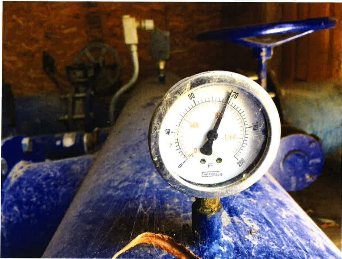
Pressure irrigation pump station discharge pressure.
