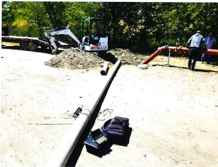
Temporary 10-inch aluminum mainline. Permanent mainline will be installed after golf season. Portable ultrasonic flow meter used for flow measurement shown on pipe.
