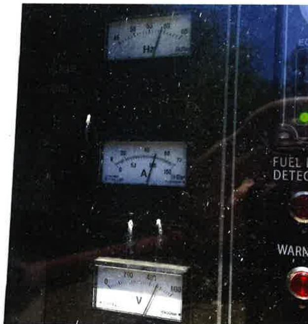
Well 2 Pump Panel. Pump is constant speed.
