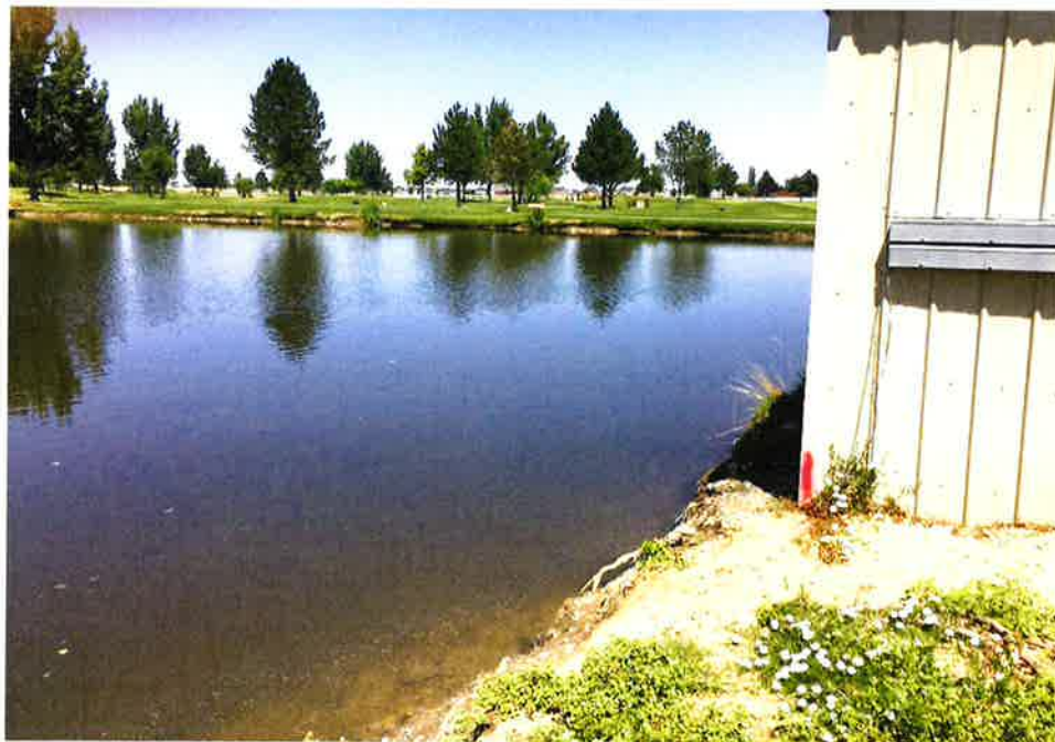
Pressure irrigation pump station (right) and pond (left) looking north-northwest. Water from Well 1 enters north side of this pond through buried pipe. Water from Well 2 enters southwest corner of pond through open channel.
