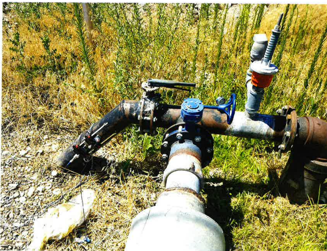
Well 1 discharge piping with portable flow meter attached
