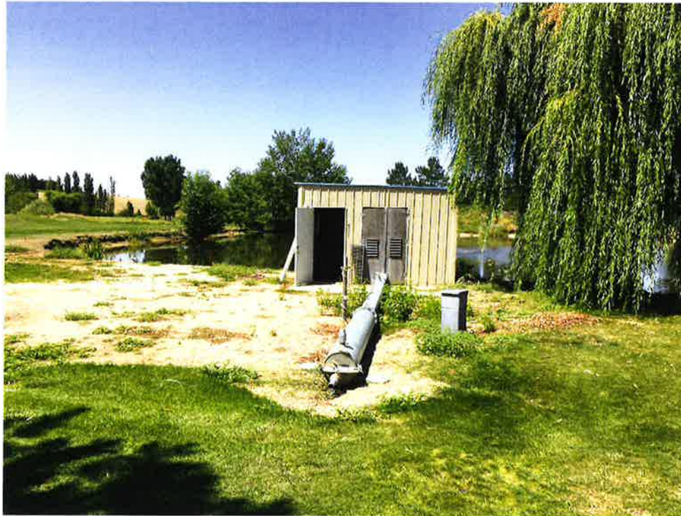
Pressure irrigation pump station with discharge pipe and filter (foreground) looking west. Water from Well 2 enters the pond through an open channel at far side of the pond.
