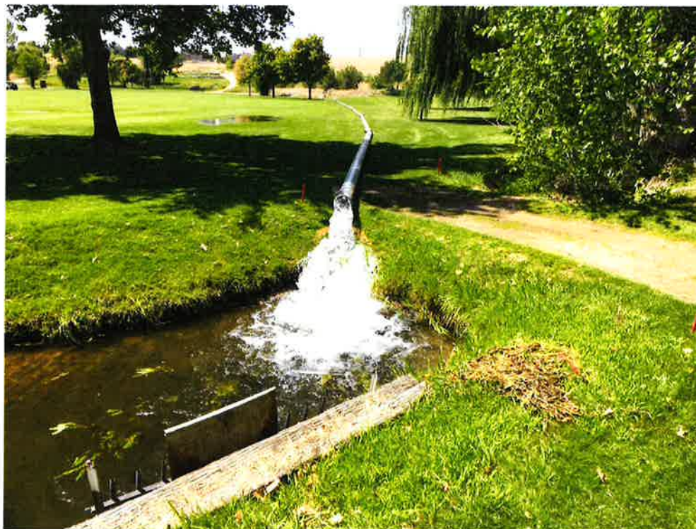
Temporary mainline discharging to golf course pond system. Headgate and trash rack to downstream ponds in foreground.
