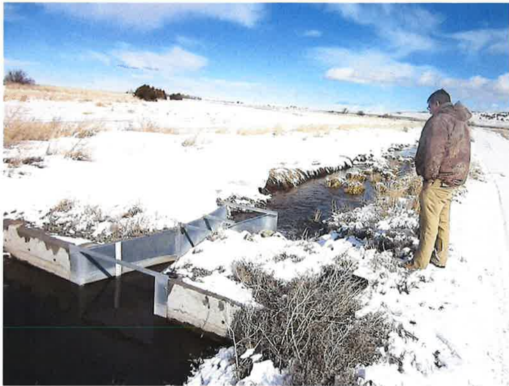
Figure 4: 18" Parshall Flume & Observer
