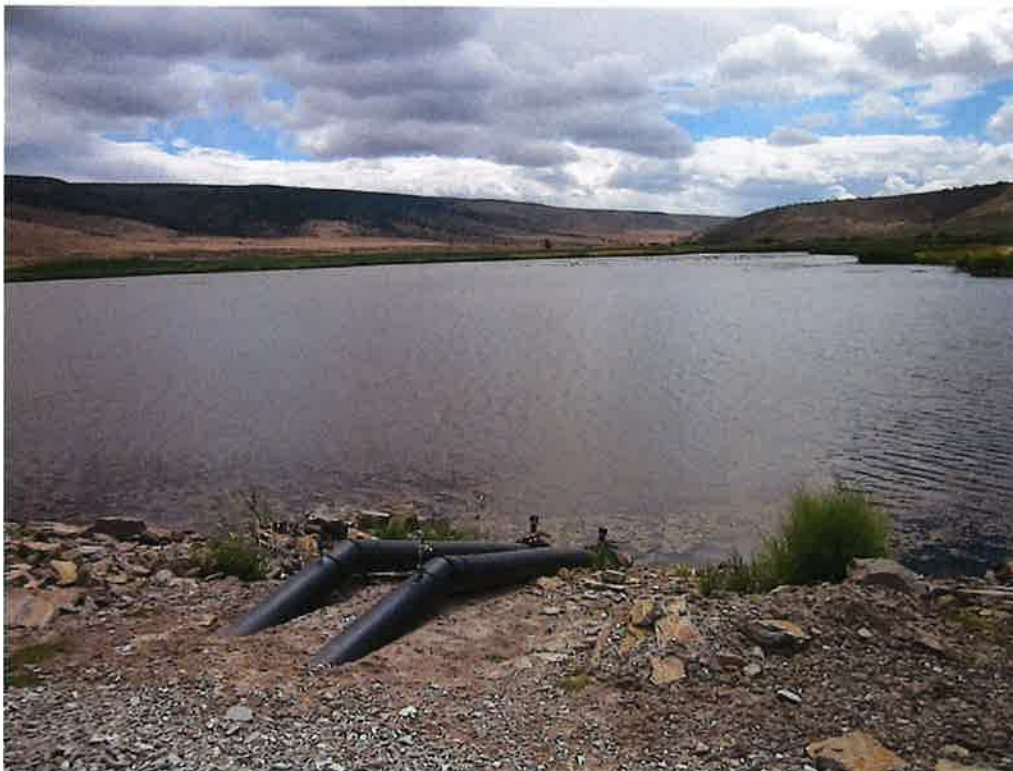
Figure 3: Intake Siphon Tubes & Reservoir
