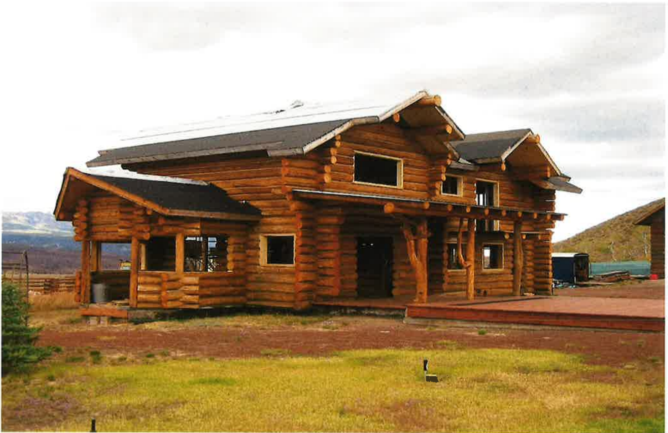
Cabin, Landscaping and Irrigation Sprinklers
