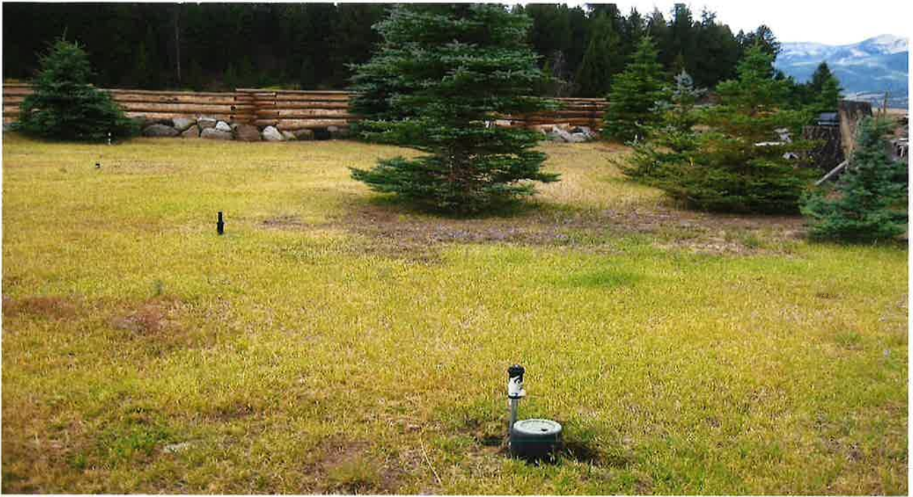
Landscaping and Irrigation Sprinklers
