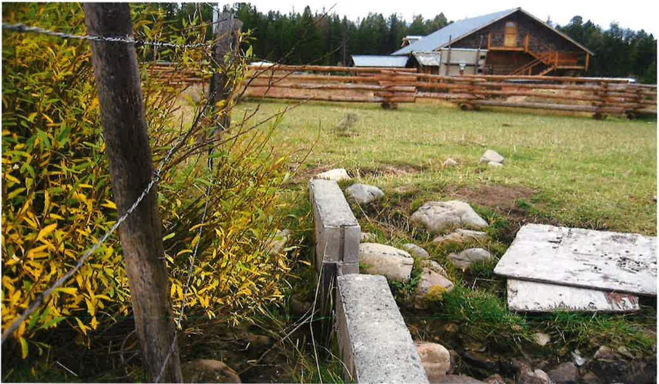
Check Gate for placement of Irrigation Pump and Hose
