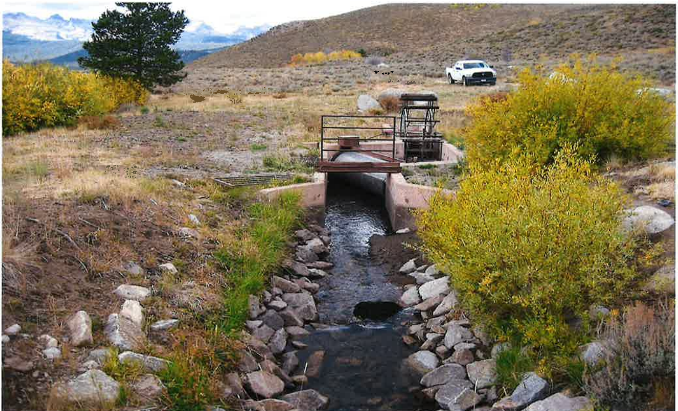
Fish & Game, fish screen in diversion ditch
