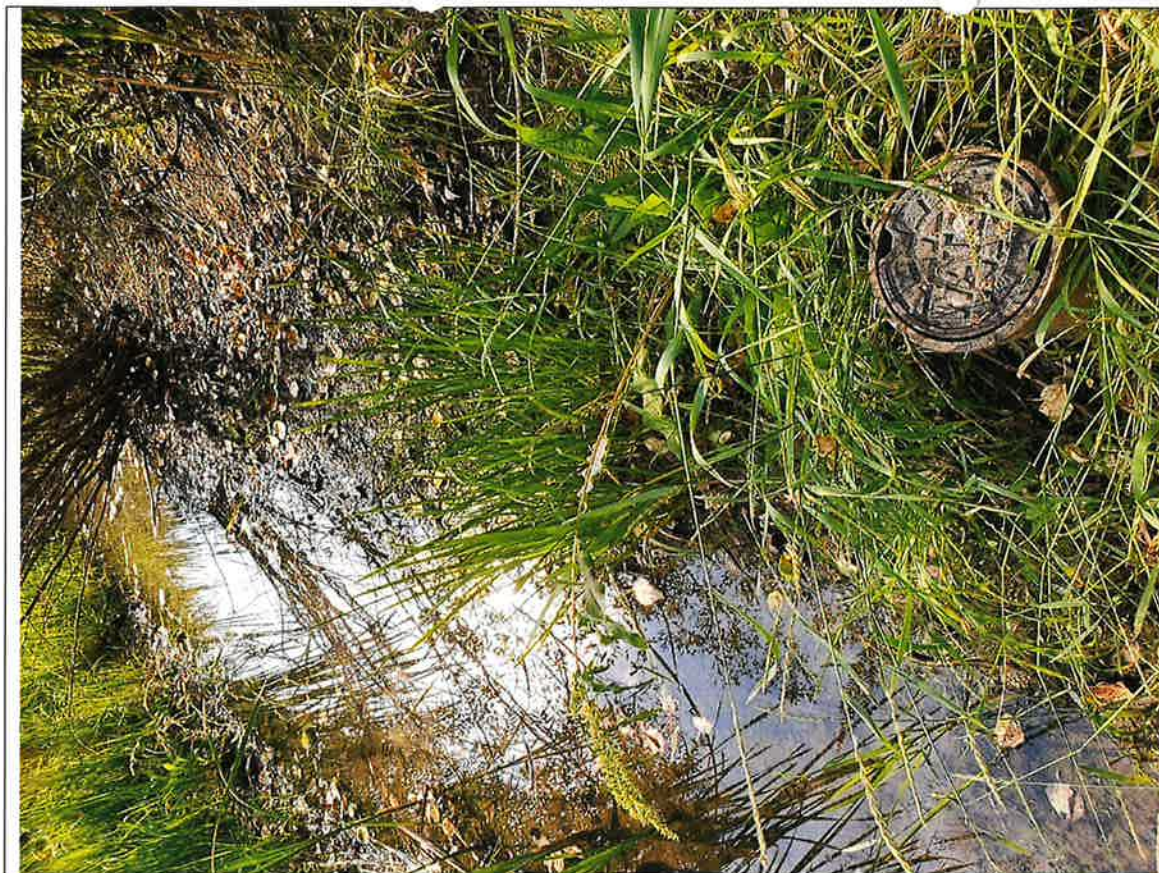
Valve used to control the release of the return water.
