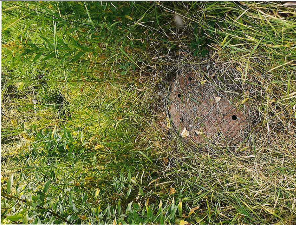
Man hole where return water is discharged into a City owned storm water infiltration basin.
