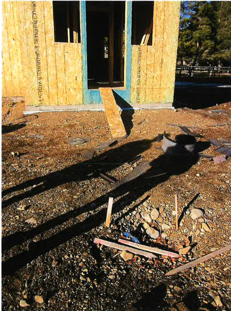
Above: Main line from well house to residence & garage near southeast corner of garage. The line forks, with one fork going to the garage and the other will go to the main residence when constructed.
