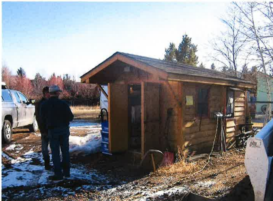
Below: Lockable well house. Photo faces south.
