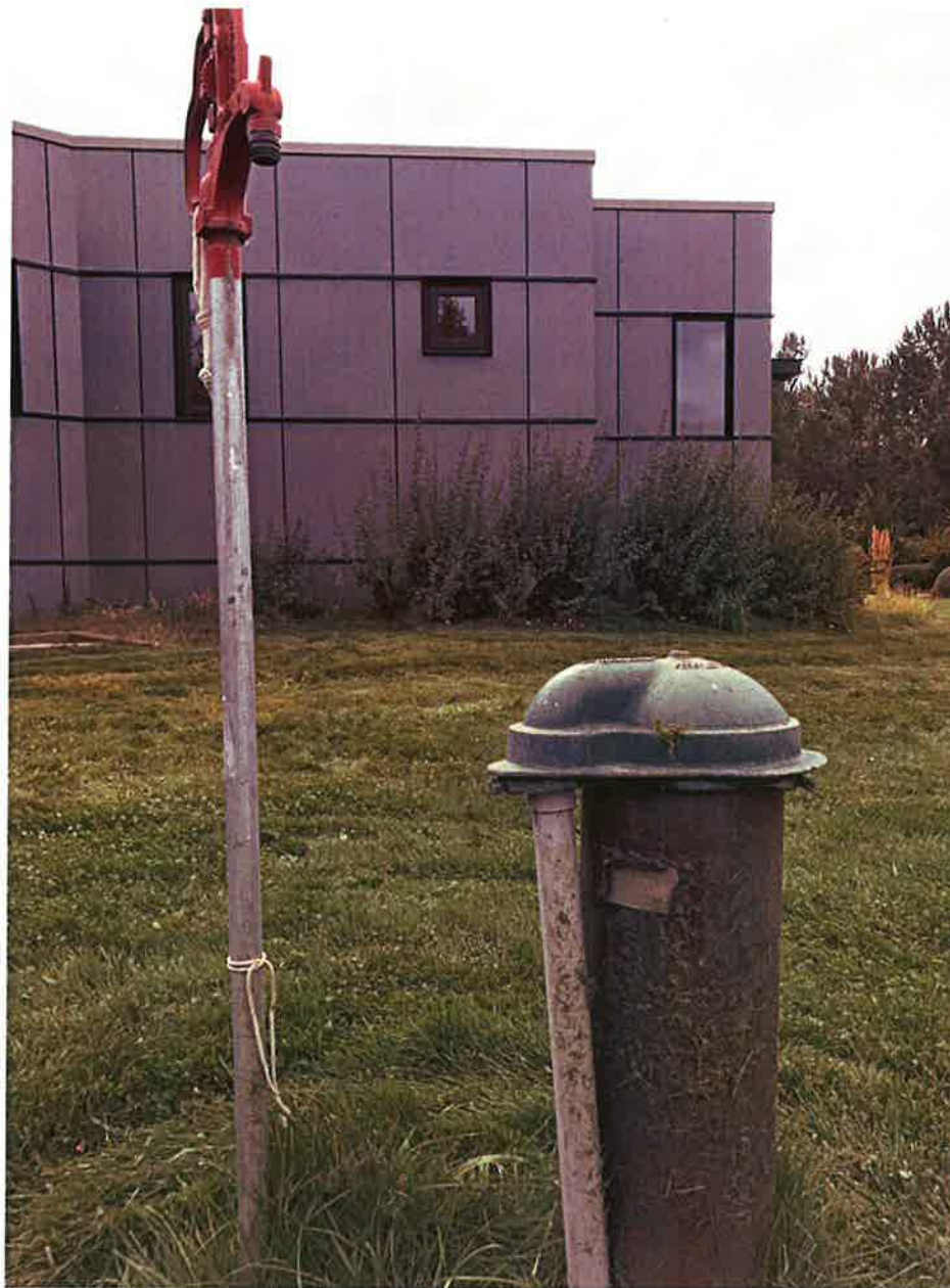
Figure 1: Wirth production well for domestic, heating and cooling uses.
