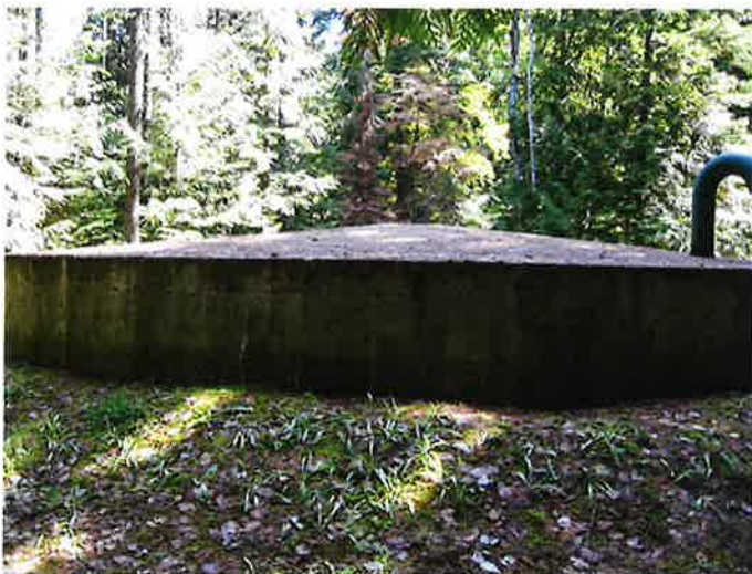
HUCK BAY Reservoir 1
