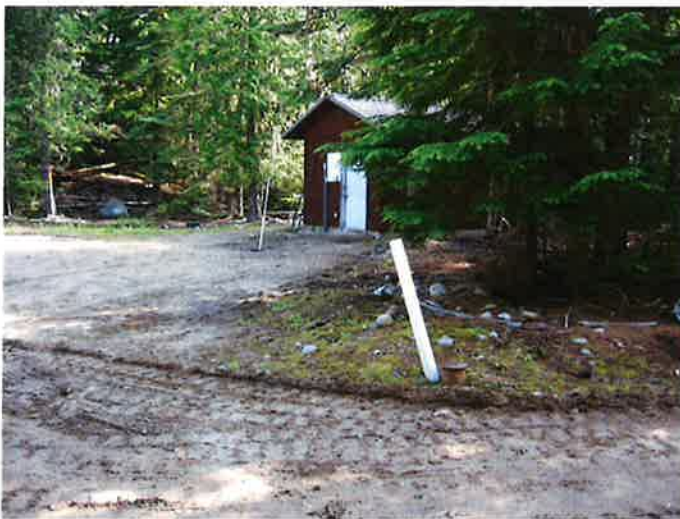
HUCK BAY Well 1 to left rear of Pumphouse
