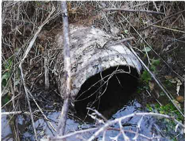
Point of Diversion (drain into ditch), beginning of reach
