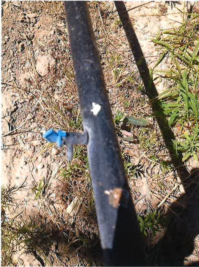
Figure 5. Drip line along the western edge of the property.
