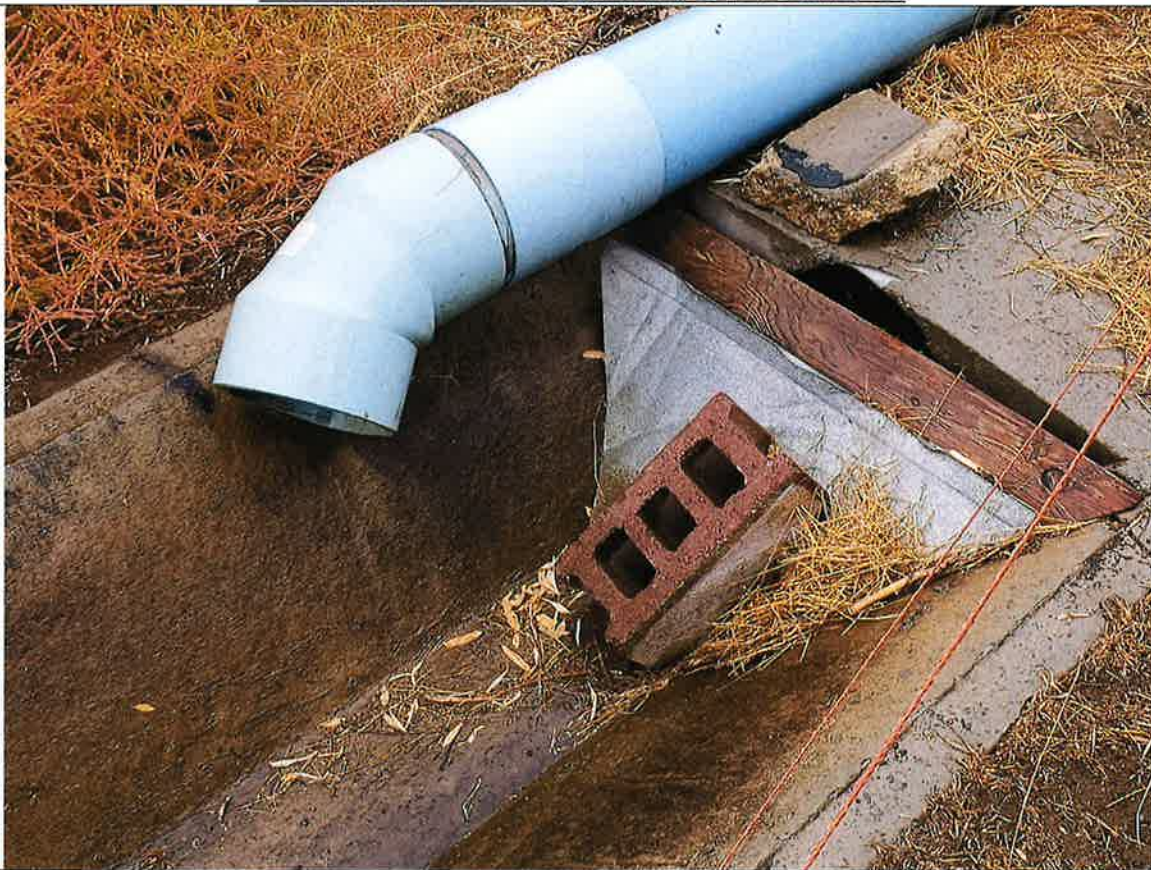
Discharge in to the concrete ditch. \frac{3}{4} inch siphon tubes are used to flood irrigate.
