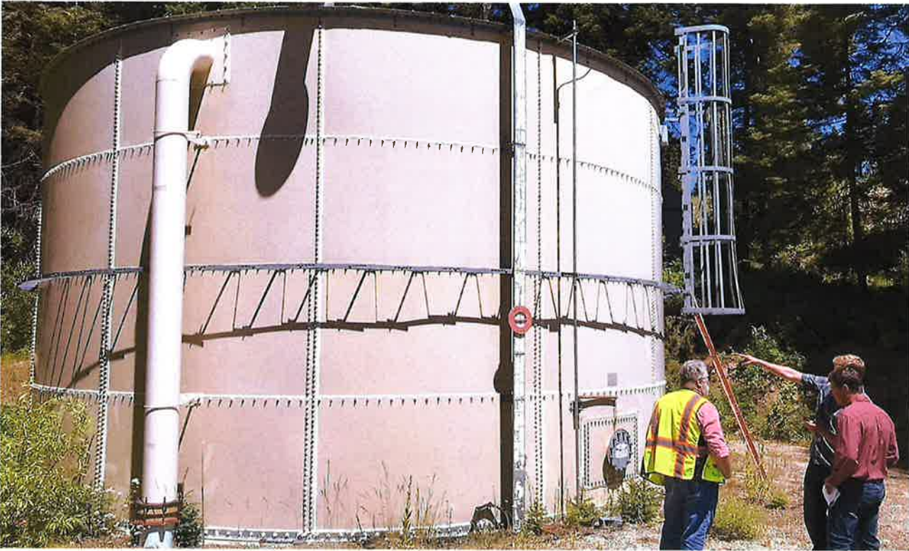
Photo 19. 32 foot diameter, 18.2 foot tall, 106,290 gallon (0.33 AF-FT) capacity tank that is associated with well 5. To measure the pumping capacity of well 5, we conducted a fill test of this tank (added a total of 1.0 feet of water). We recorded the water level over time, which allowed us to calculate the volume over time.
