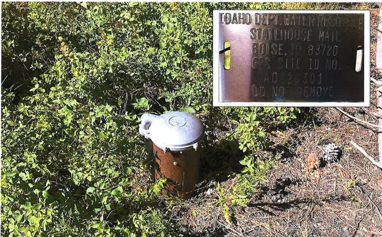
Photo 4. Well 9, also known as the Batch Plant Well, was used during construction activities. The well did not have a tag number. We added well Tag A0020301 to the well during the field exam. The well log indicates that the well tag issued for this well was D0038096.
