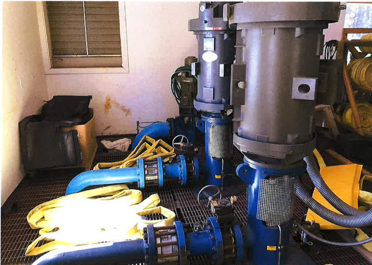
Photo 18. Wet well associated with water from well 5. Water from the adjacent 106,290 gallon steel tank fills the wet where it is prepared for snowmaking during the winter months. The wet well is not used to irrigate the golf course.
