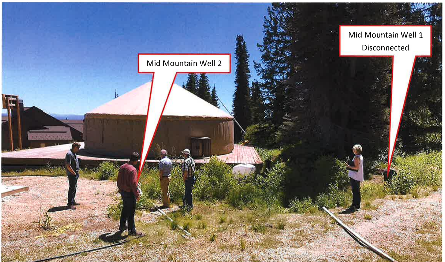
Photo 22. Mid Mountain Well 1 (disconnected, but not abandoned) and Mid Mountain Well 2 (operational). Construction of the Mid Mountain Tamarack lodge is mostly complete, but was never put into service. The water supply infrastructure was put into place before the project was abandoned during the economic downturn around 2008. Water from Mid Mountain Well 2 was going to be pumped into three (3) 2,100 gallon tanks located in the basement of the lodge. The well is operational and water from this well is used for incidental needs for the adjacent yurt and other low volume activities. We measured the well capacity with a 5 gallon bucket and stopwatch during the field exam (15.8 gallons per minute; 0.035 cfs).
