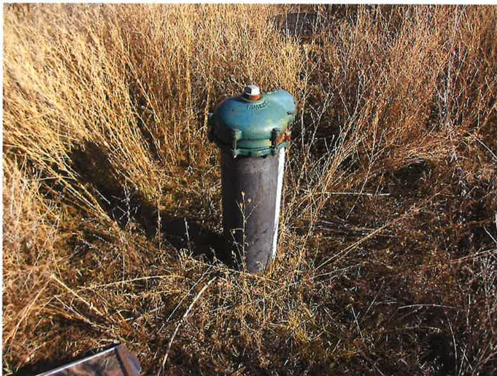
Well #1 - Primary well, off-site
