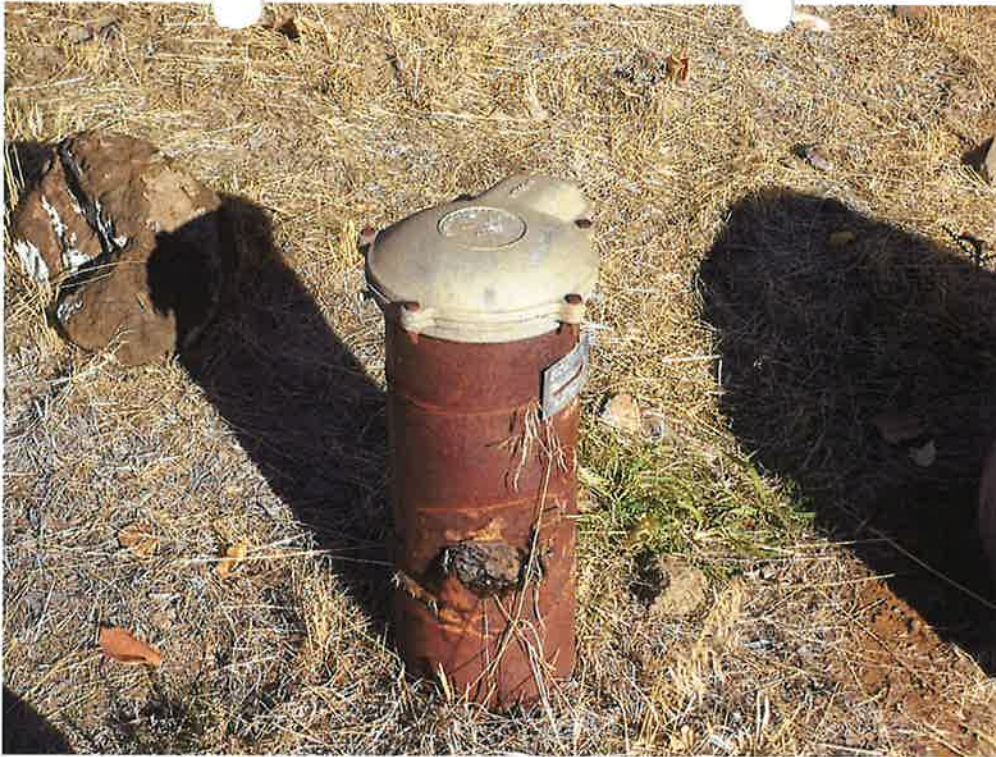
Well #2 - Backup well, on First Fruits property
