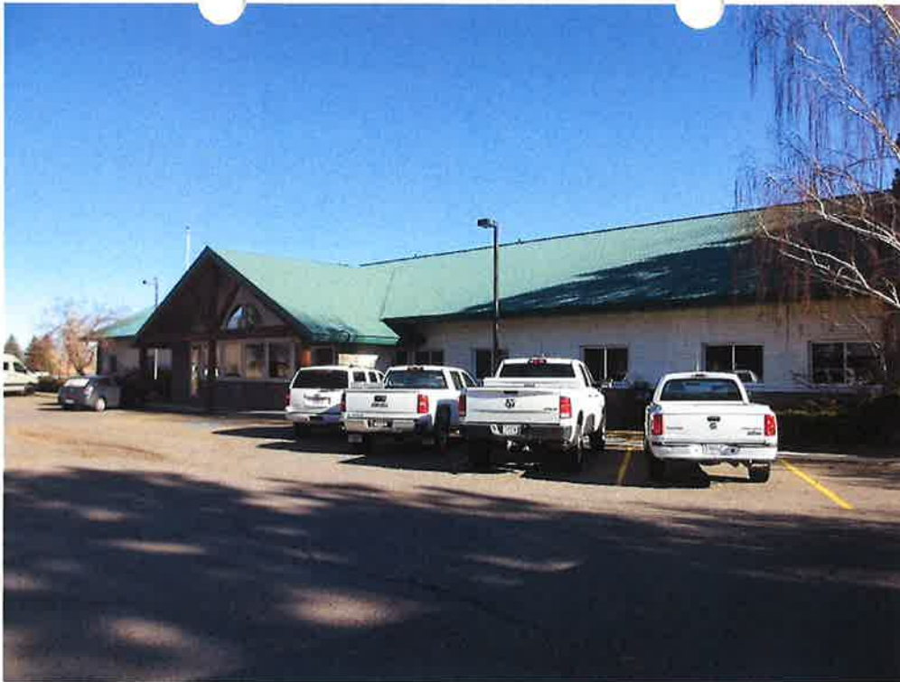
Front view of Forest Service building
