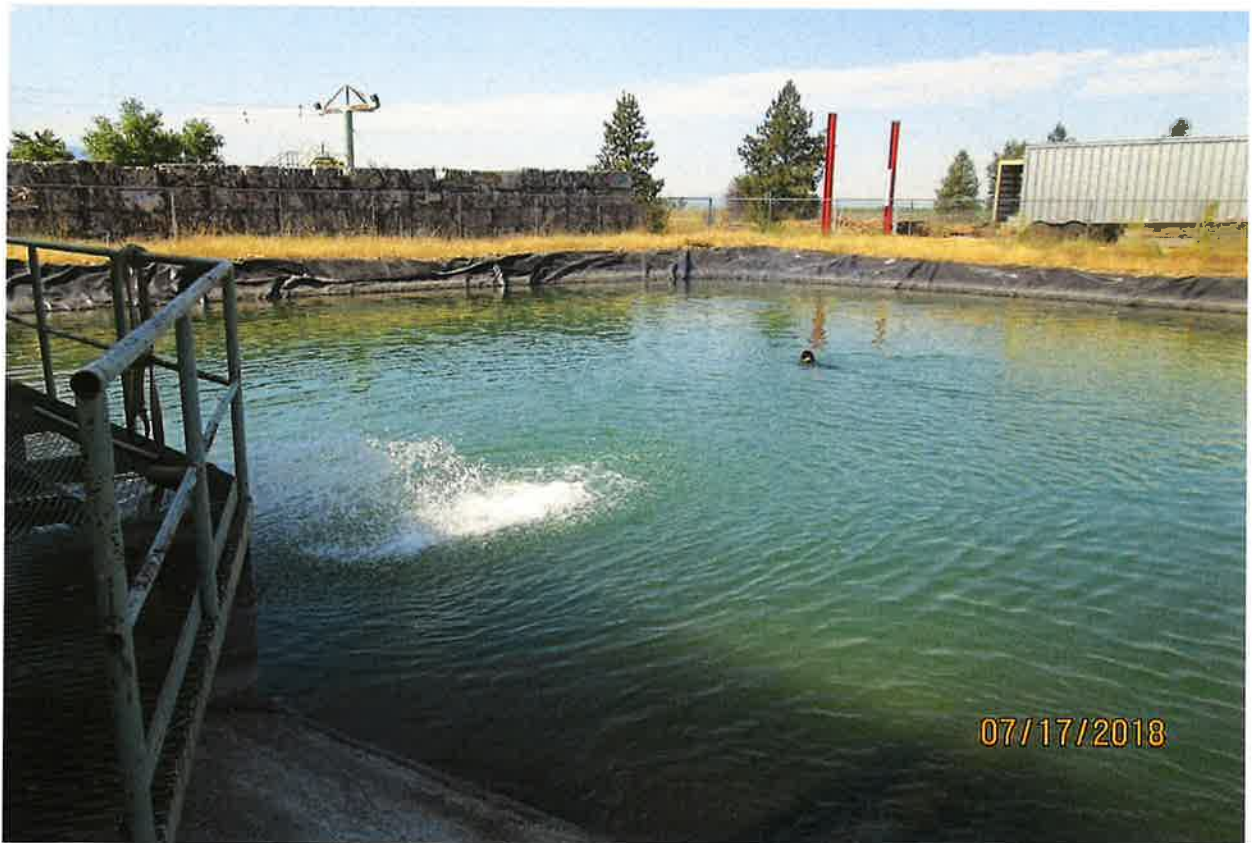
Fire protection storage.
