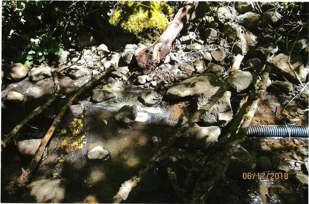
Point of diversion.
