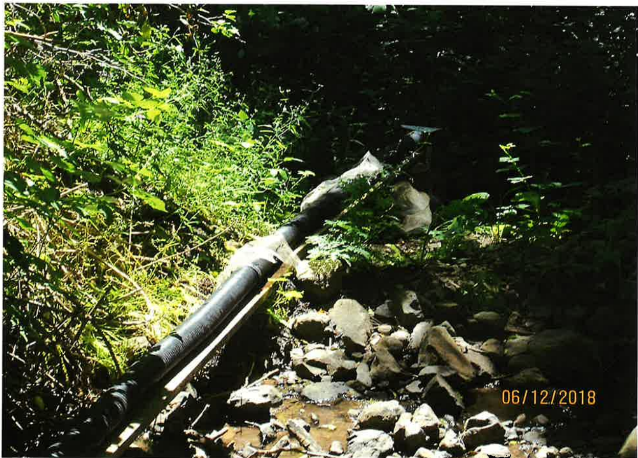
From point of diversion it went to 5 gallon bucket with line for irrigation.
