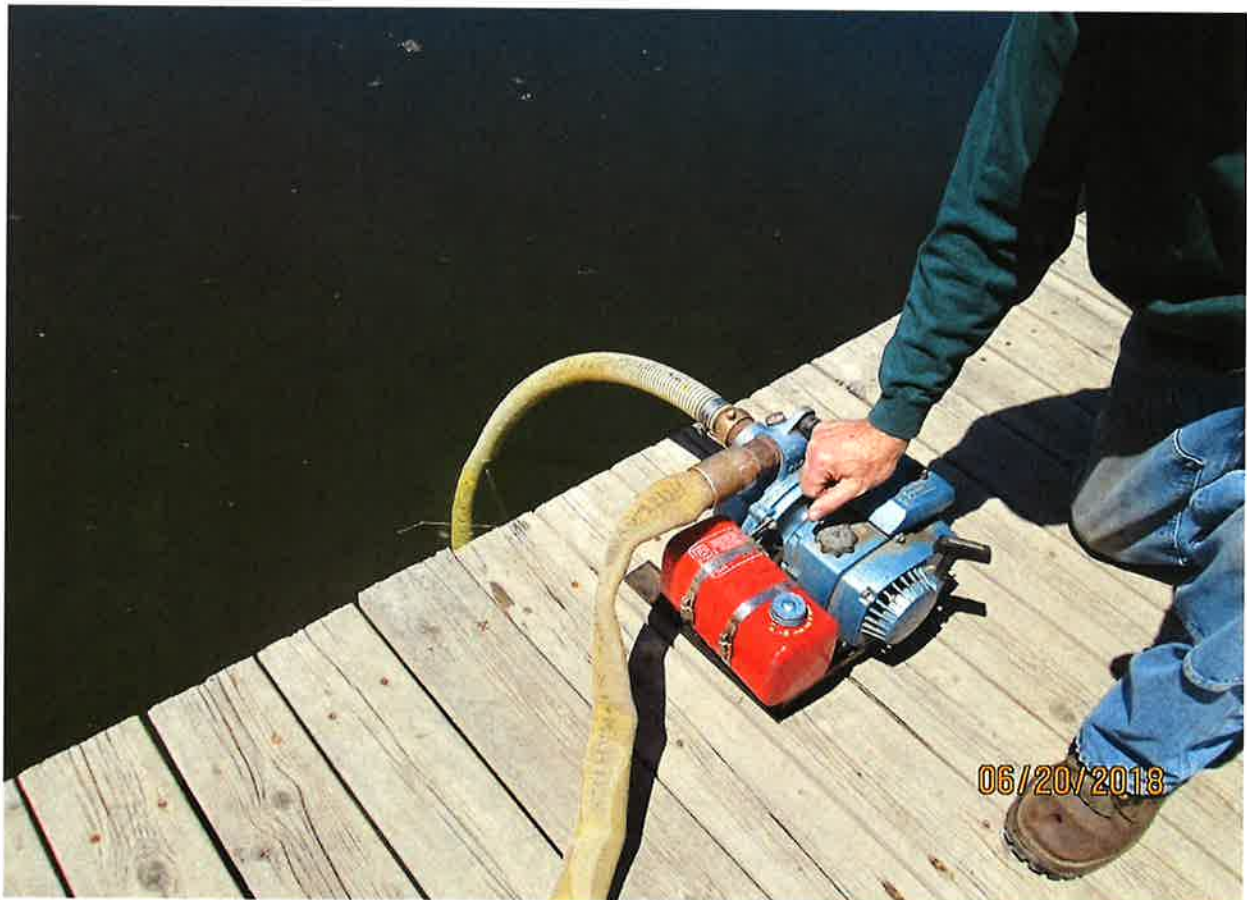
Applicant had very old pump with unknown horsepower.
