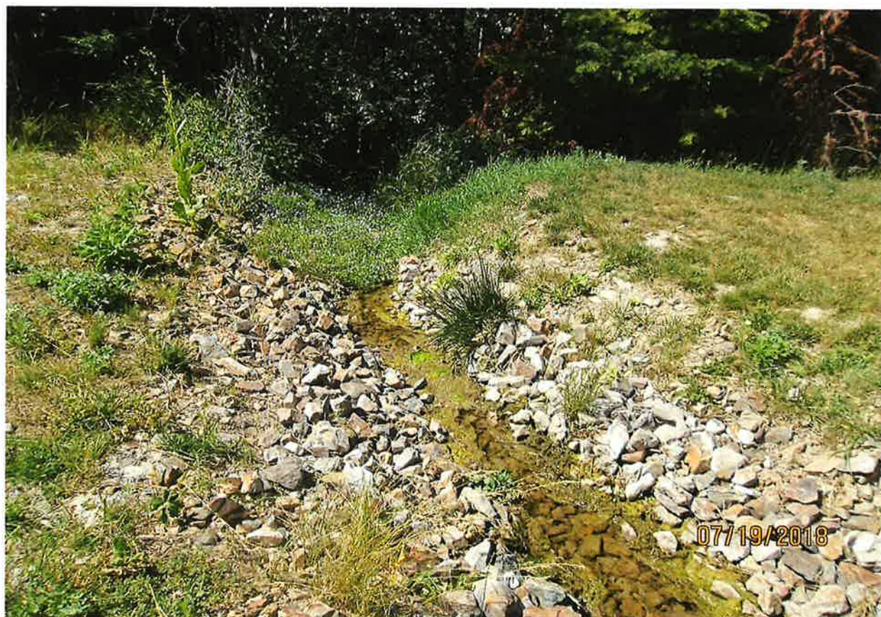
Overflow channel looking downstream of dam.
