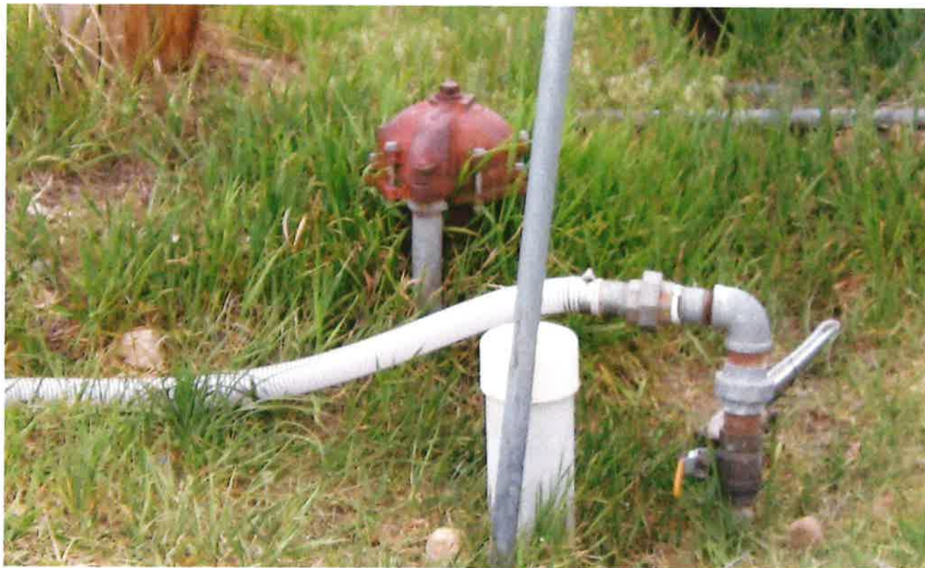
Well Head and Irrigation System Connection
