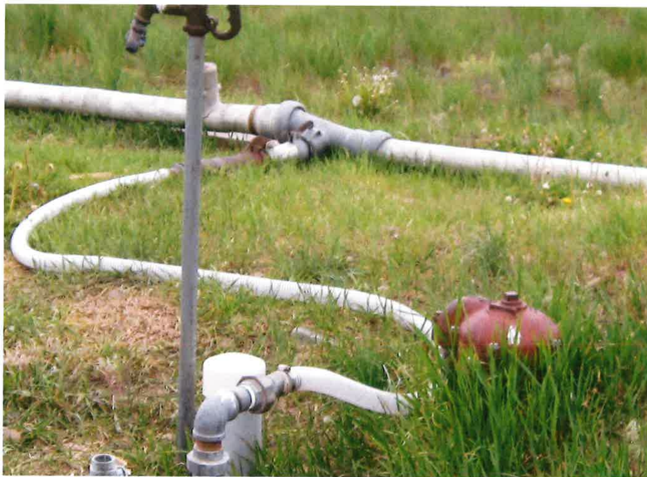
Well Head and Irrigation System Connection
