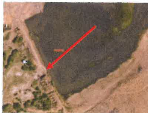
2017 imagery with breach visible.
