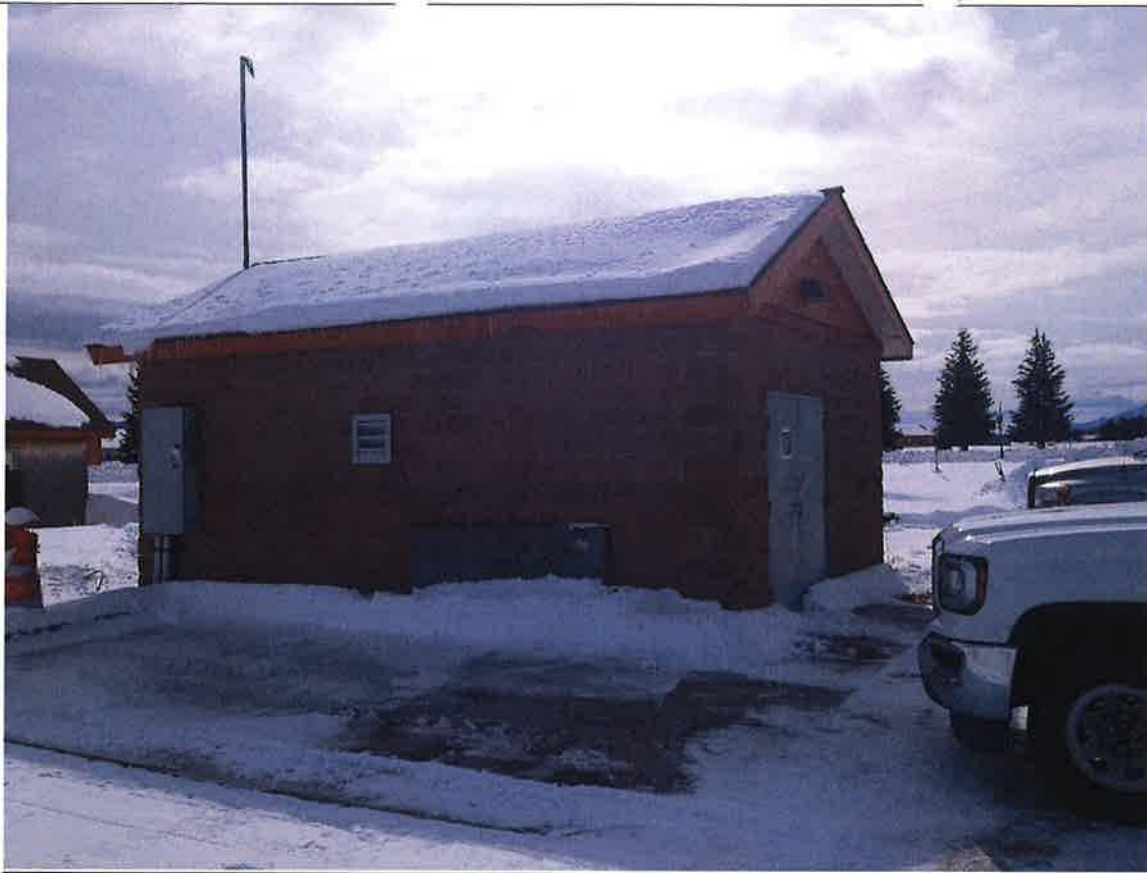
Well House #2 located at the corner of W Roseberry Road and Schultz Lane.
