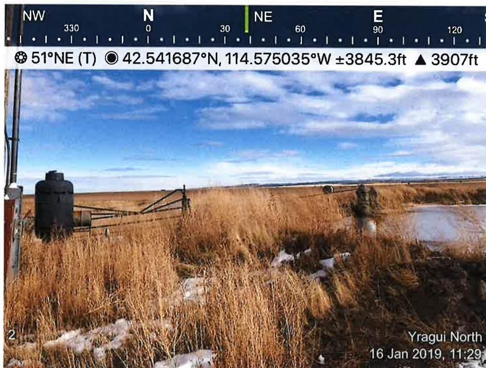
Figure 2: POD; lift pumps and irrigation pond
