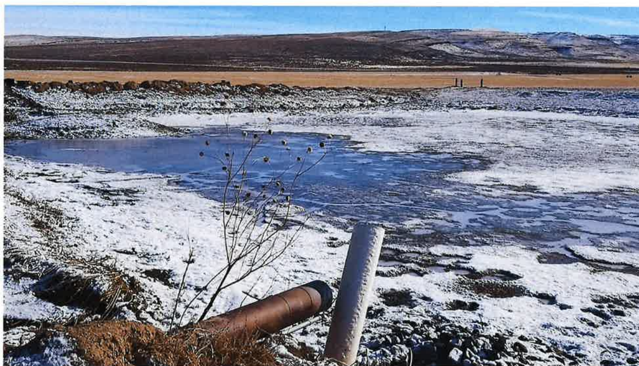
Figure 3: Outlet of pipe from well and irrigation/stockwater pond
