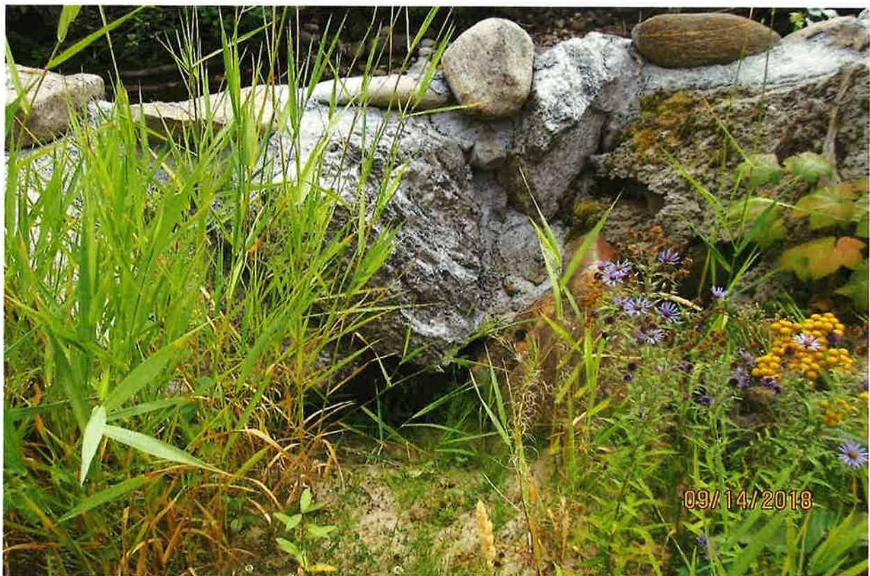
10 inch pipe on inside of diversion wall. Water not diverted at time of exam due to sand in settling pool.
