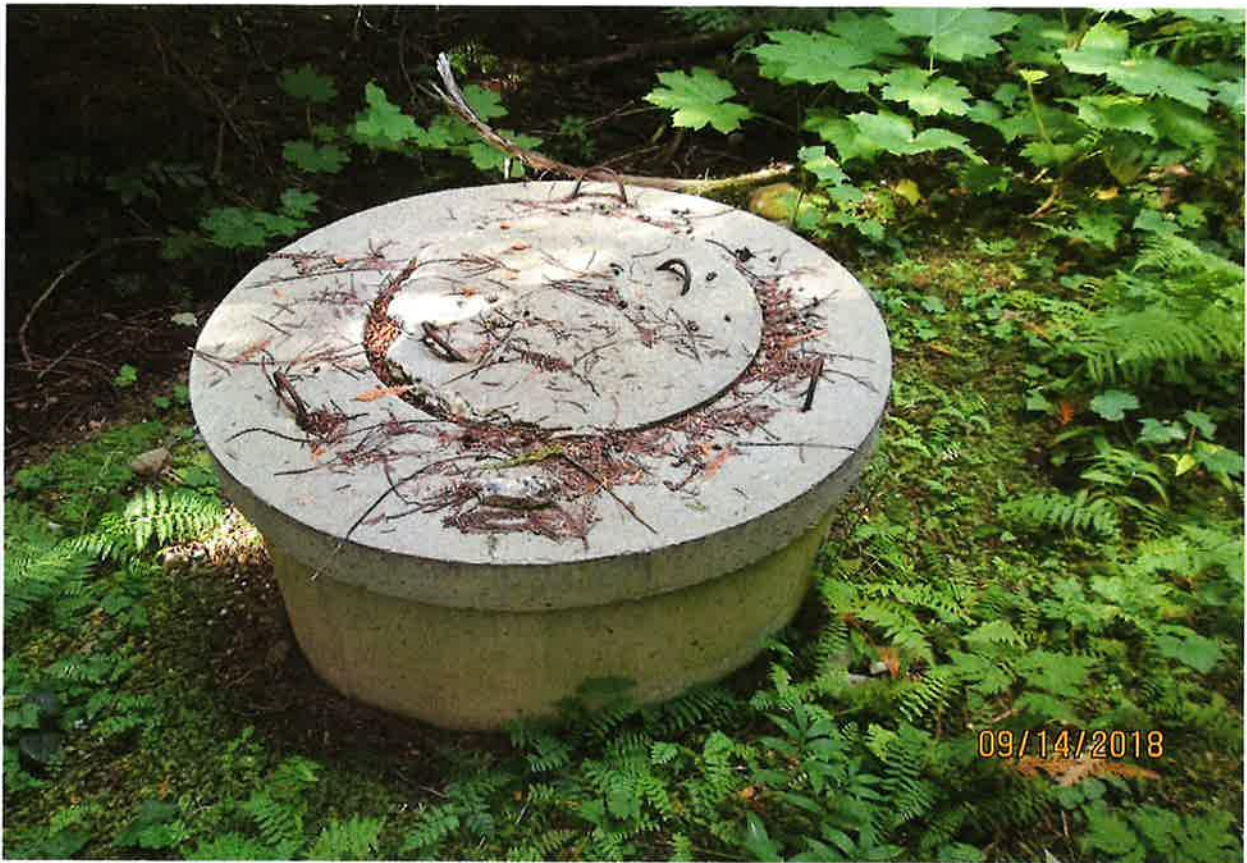
Point of diversion.
