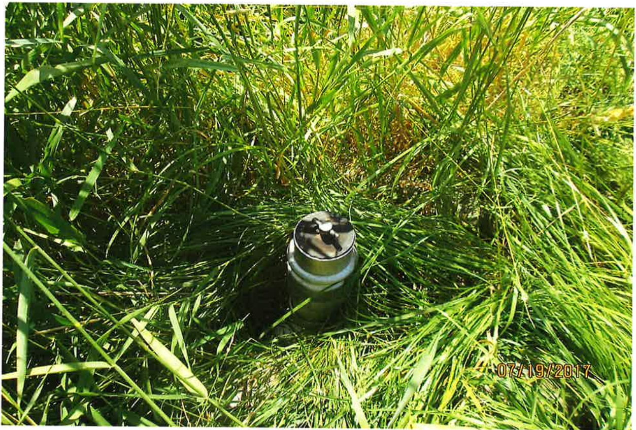
Riser on the creek bank next to point of diversion.
