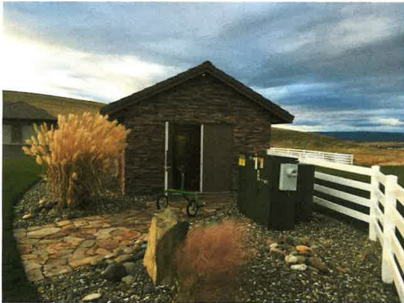
COMPLETED WELL HOUSE
