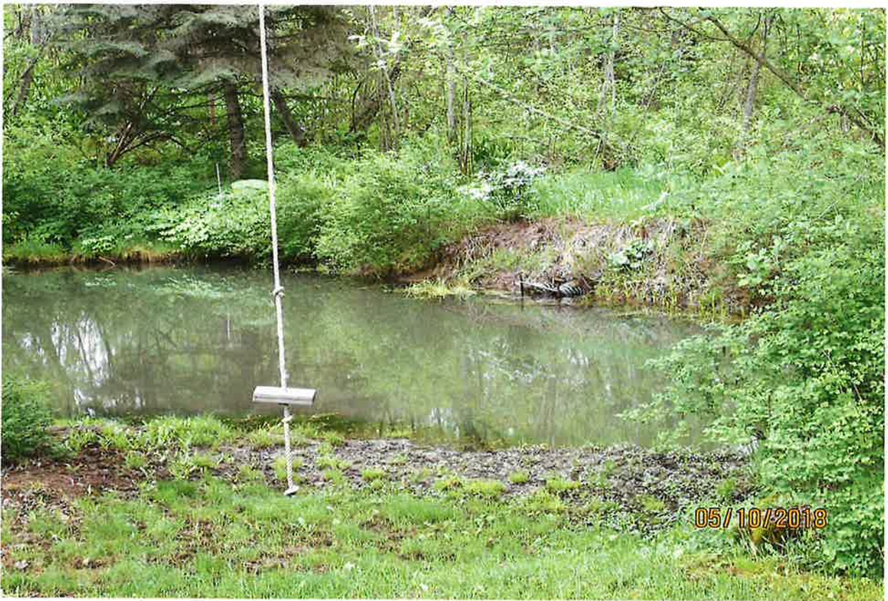
Storage place of use and culverts returning flow back to creek.
