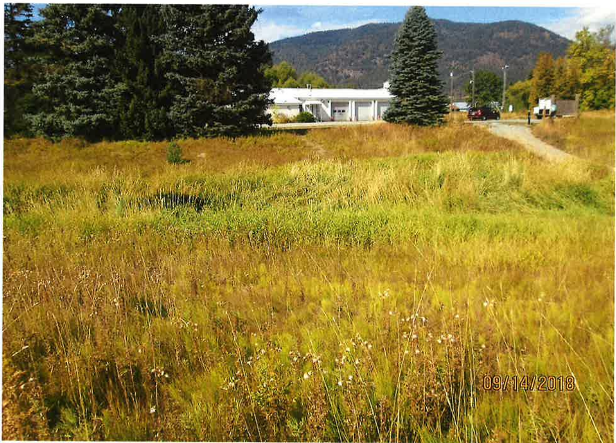
Upper end of pond filled with grass because of no maintenance.
