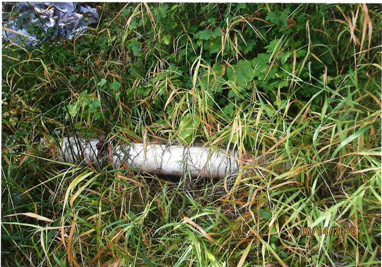
Pipeline going uphill to place of use.
