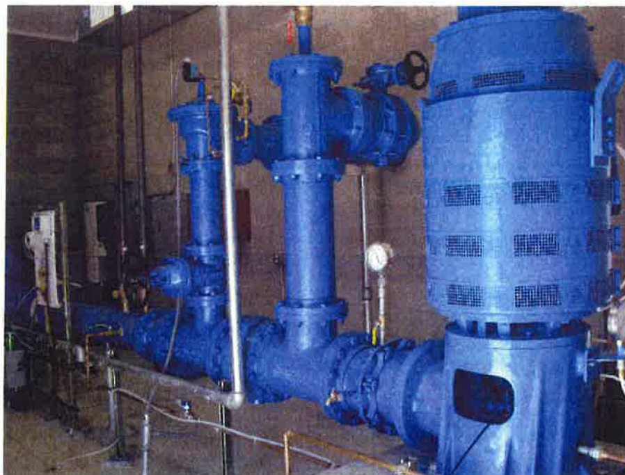
Figure 6. Diversion Works, Looking Northwest
