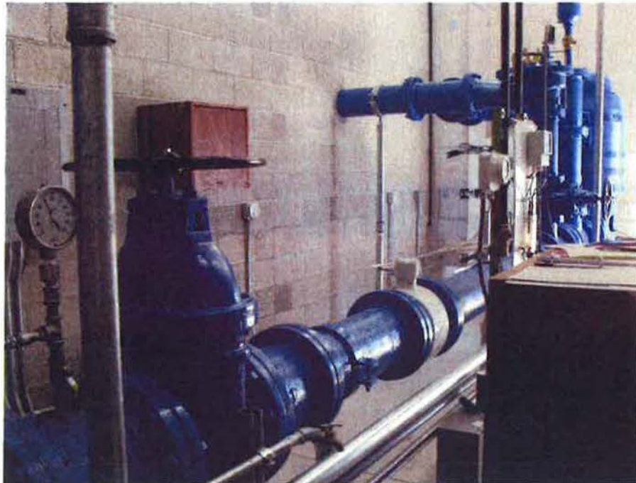
Figure 7. Diversion Works, Looking Northeast
