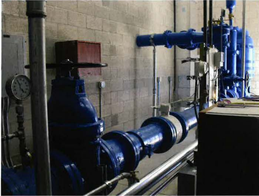
Figure 7. Diversion Works, Looking Northeast
