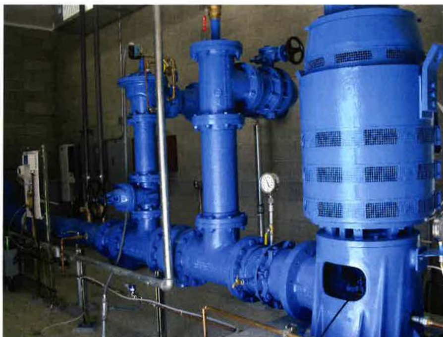
Figure 6. Diversion Works, Looking Northwest
