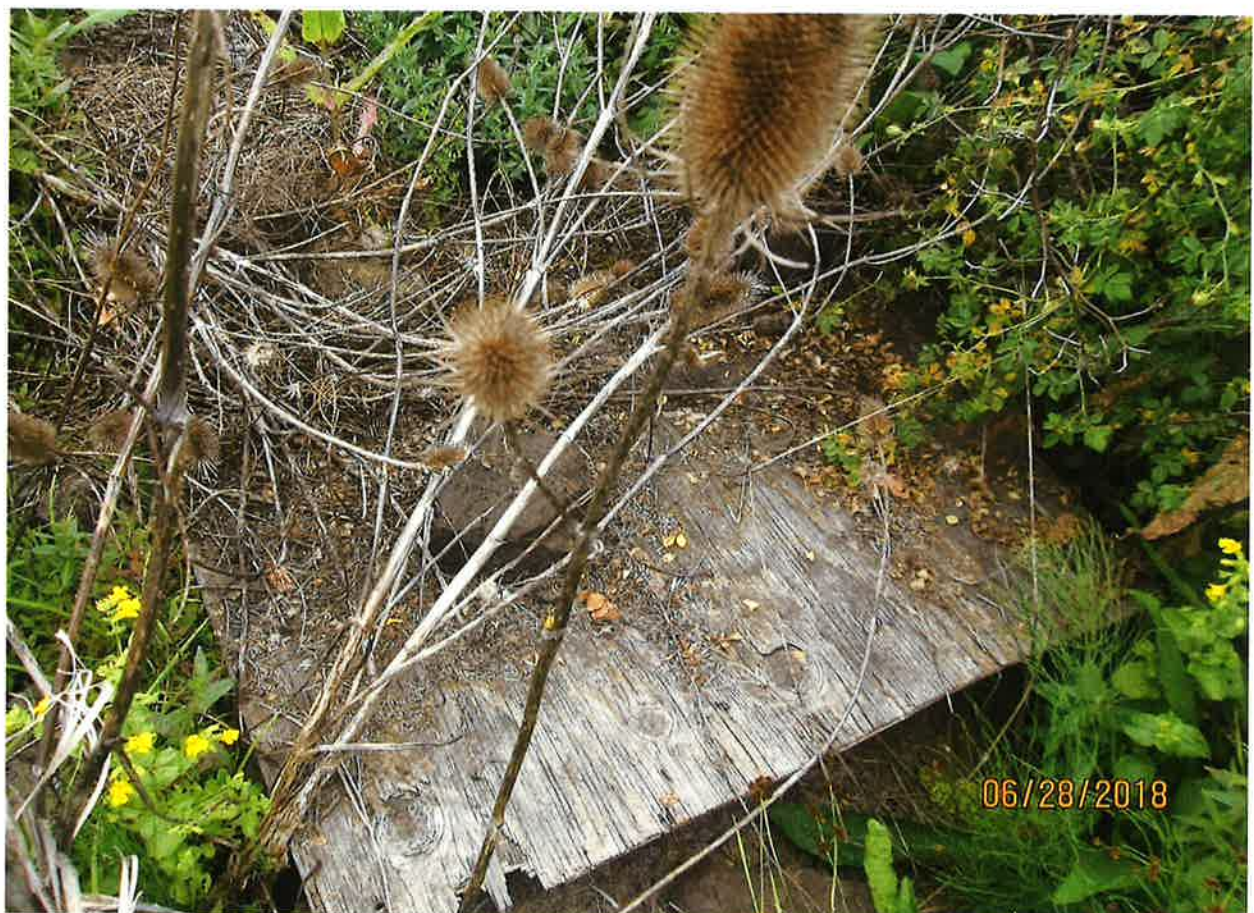
Point of diversion. Culvert dug into ground with small unknown pump inside.
