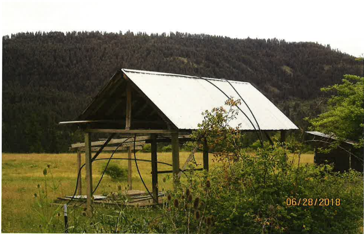
Poly pipe that owner would use to gravity flood irrigate areas below point of diversion.
