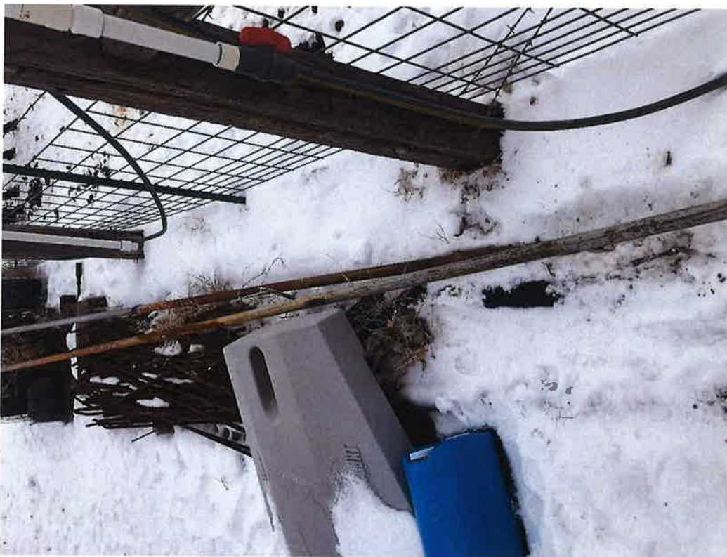
Figure 8. (con't) Pump and riser pipe recently removed from Schvaneveldt well.
