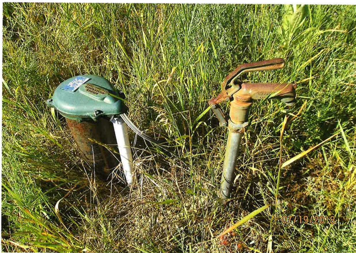
Frost free hydrant where 5 gallon bucket test was performed and filled in 8 seconds.
