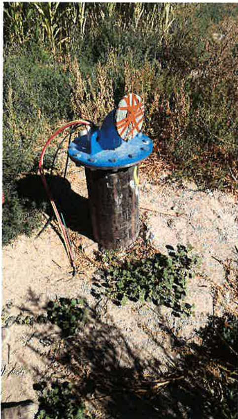
Figure 3 The three secondary wells located at the POU and used as a backup.
