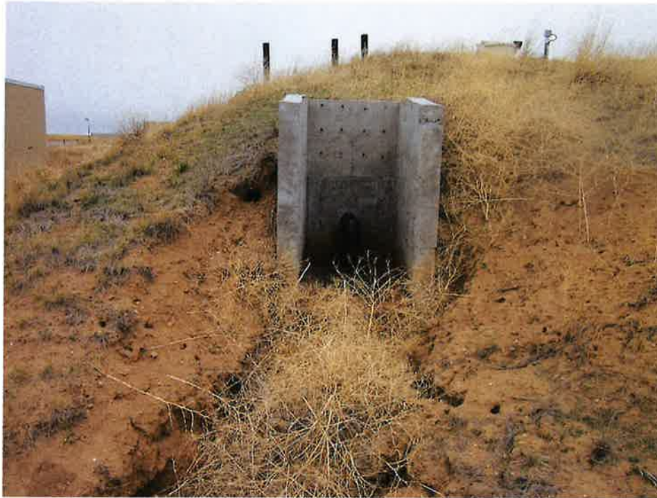
Figure 3: Drain on east side of storage tank
