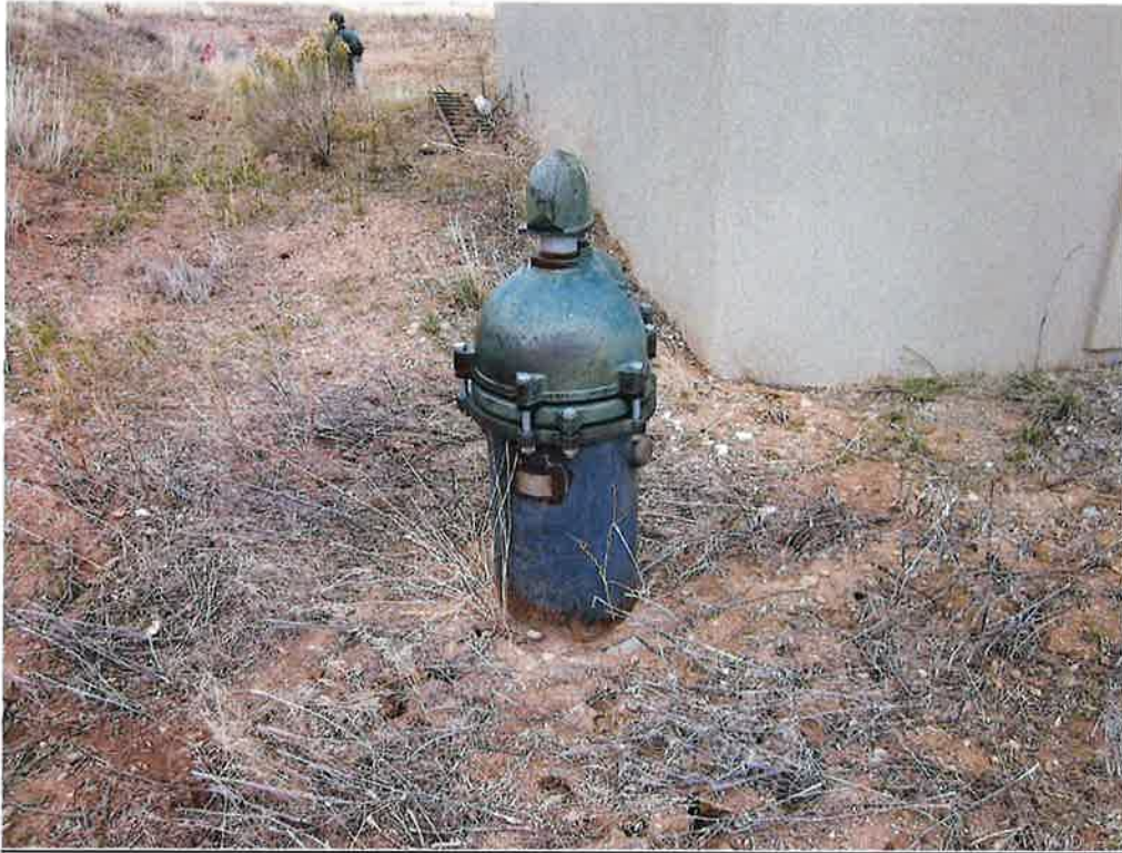
Figure 1: Backup well looking east to primary well
